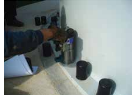
Foundation bolt tensioning
