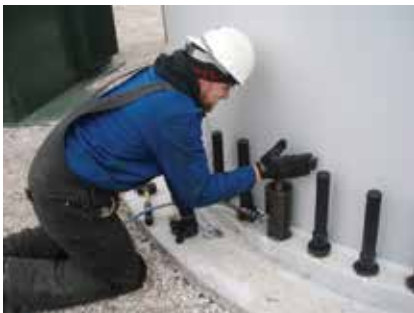
Foundation bolt tensioning
