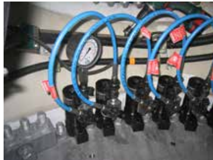
Tower bolt tensioning
